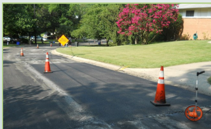
Example of completed patching
