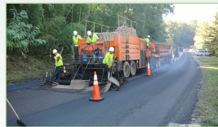
Typical micro-surfacing operation
