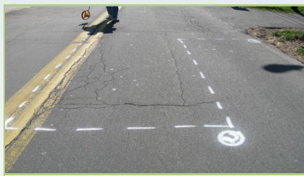
Typical survey paint markings
